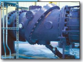
Tilted Disc<sup>®</sup> Check Valve with Bottom Mounted Oil Dashpot.
