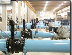
Tilted Disc<sup>®</sup> Check Valve with Top Mounted Oil Dashpot.
