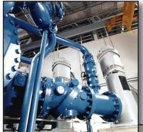
Tilted Disc<sup>®</sup> Check Valve with Well Service Air Valve on Vertical Turbine Pump.
