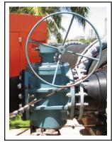
Cam-Centric<sup>®</sup> Plug Valve with worm gear actuator
