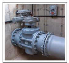
Cam-Centric<sup>®</sup> Plug Valve with motor actuator
