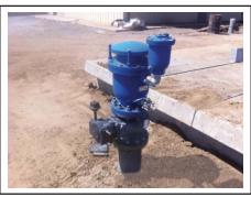
Cam-Centric<sup>®</sup> Plug Valve with Val-Matic dual body combination Alr Valve
