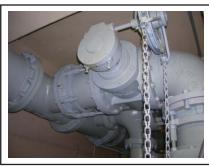
Cam-Centric<sup>®</sup> Plug Valve with worm gear actuator and chainwheel
