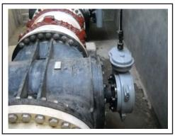
Cam-Centric<sup>®</sup> Plug Valve with worm gear actuator and extension stem
